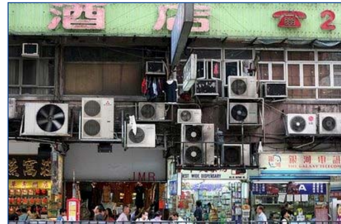
Air Conditioners in Beijing, China
