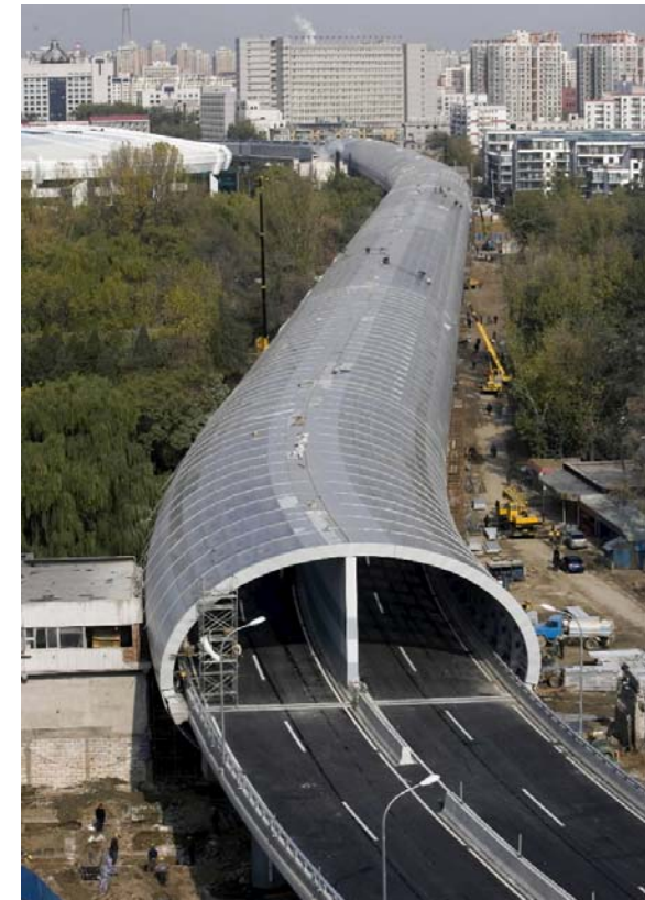
Zhanxi bridge highway, Beijing China
